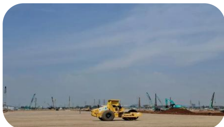
Early site preparation
