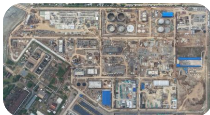
Major structure &amp; infrastructure in place
